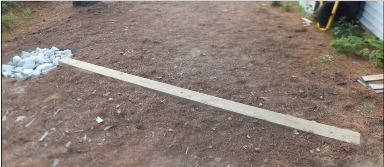
A simple timber waterbar directs water off to the left of the trail. Piles of stones help slow water flow to prevent downslope erosion. Photo Credit: Acton Wakefield Watersheds Alliance ( awwatersheds.org ).
