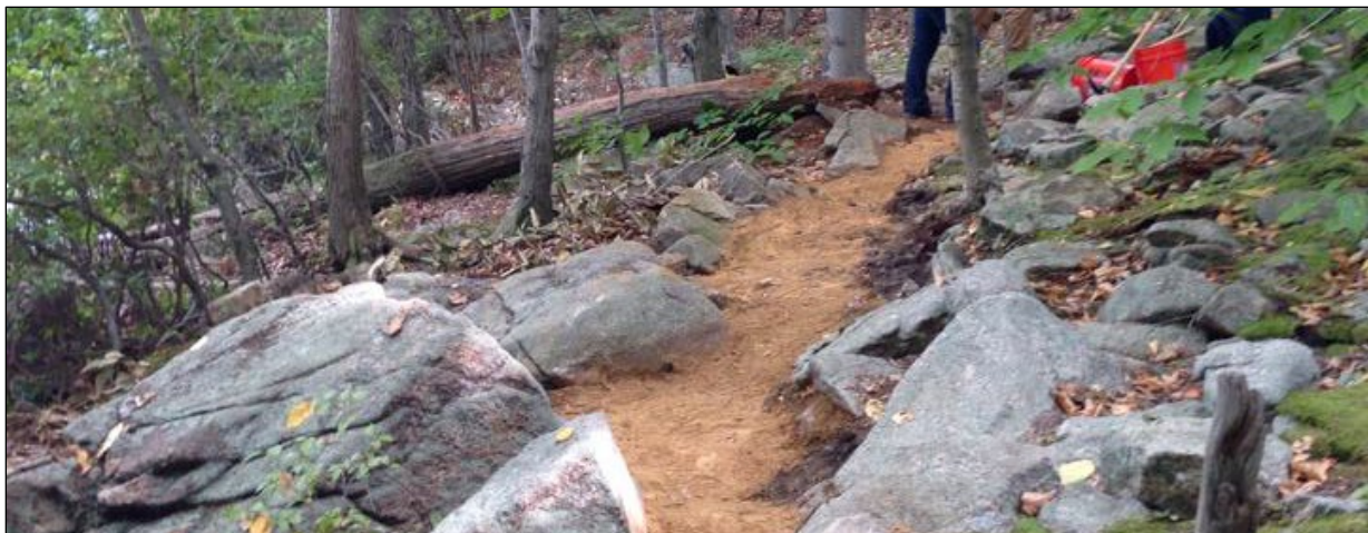
A natural-surface trail, with the “peanut-butter” color of the trail tread coming from local mineral soil compacted into a firm walking surface.
