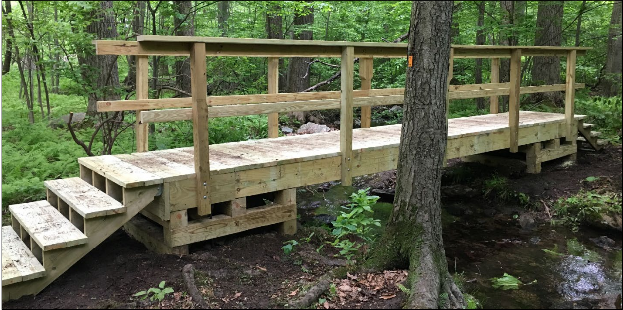
A classic wooden trail footbridge built in the simple "box bridge" style by an Eagle Scout. This location is inaccessible to vehicles and mechanized equipment, so all materials had to be carried to the location piece by piece.
