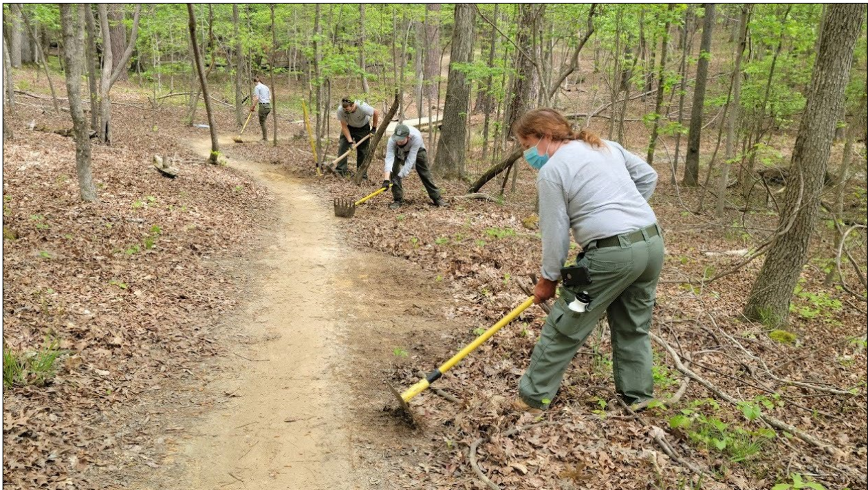
Volunteers de-berming the outer edge of a trail by dragging away accumulated material.
