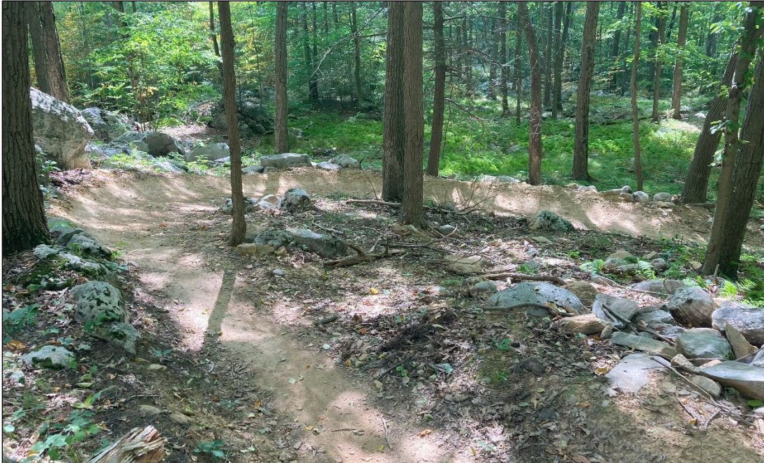
View from the top of a climbing turn. Note that this turn is designed for use by mountain bikers as well as hikers, so it features a banked berm that allows bicyclists to safely turn with it while maintaining momentum.
