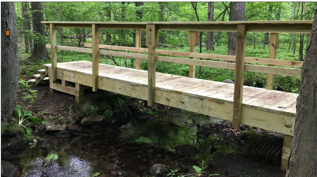
The same bridge, seen from the opposite bank. This style is considered the standard for bridges in the 15'-25' range.
