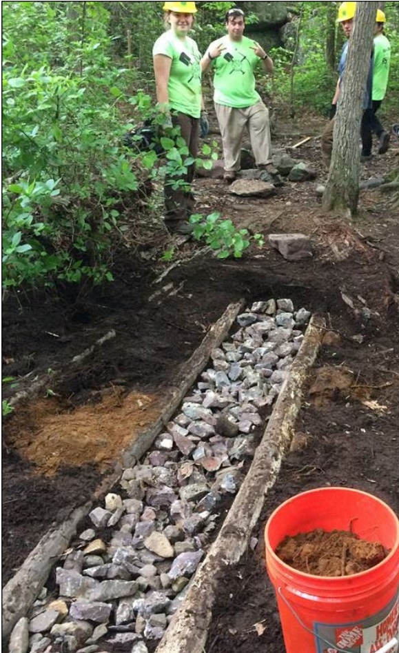
Timber turnpike with a base of stone crush fill.
