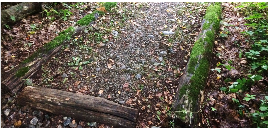
Even when the timber grows old and weathered, turnpikes usually continue to function as intended with little maintenance.
