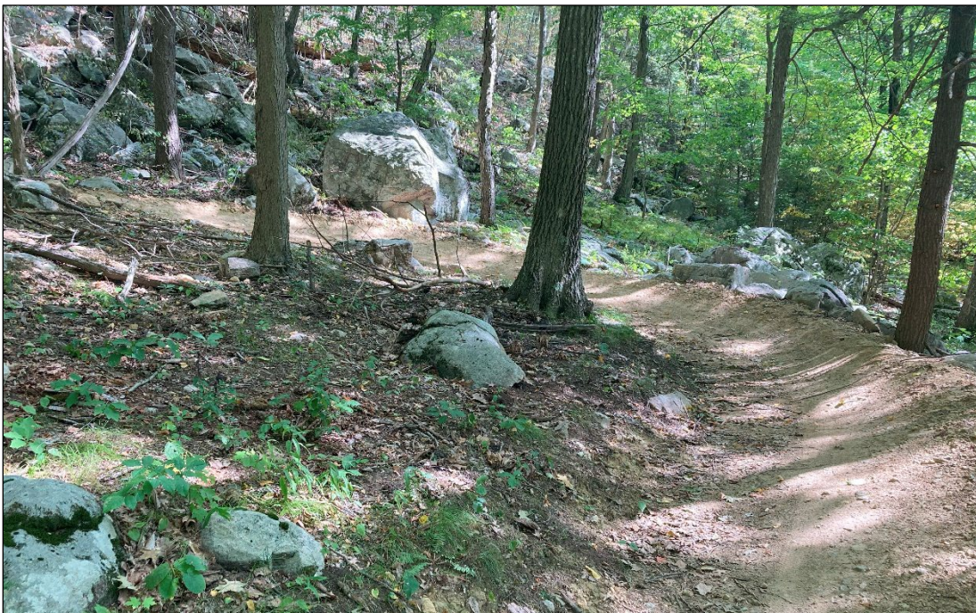
View from the bottom of the same climbing turn. Because of the banked berm, this turn will trap and channel water down the trail. For this reason, a grade reversal exists right behind the photographer's position to shed water as soon as possible.
