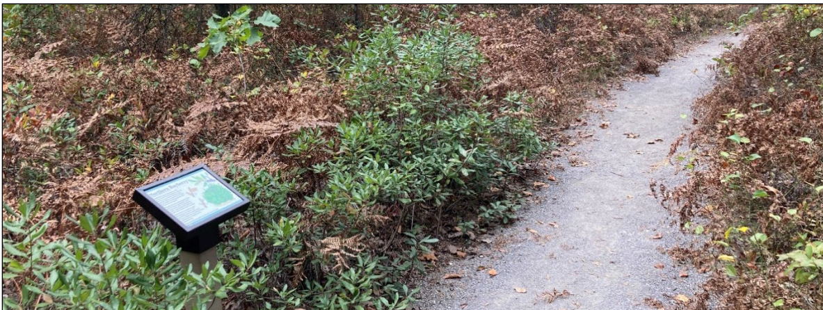
Crushed stone surfacing is an absolutely essential part of many accessible trails.
