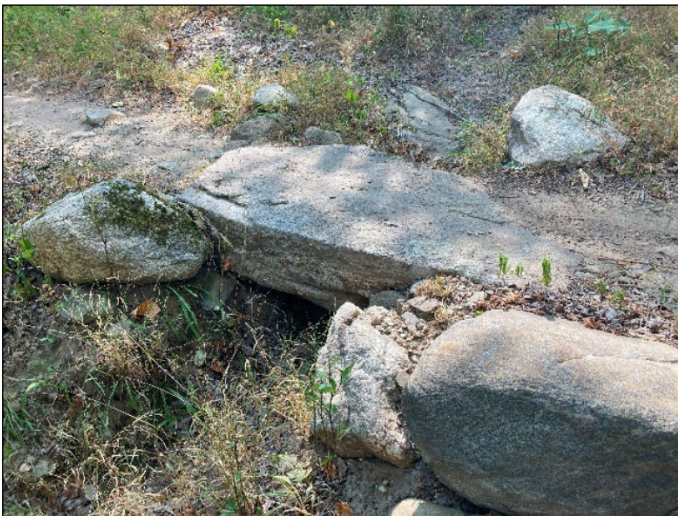
Closed culvert with single stone on top.
