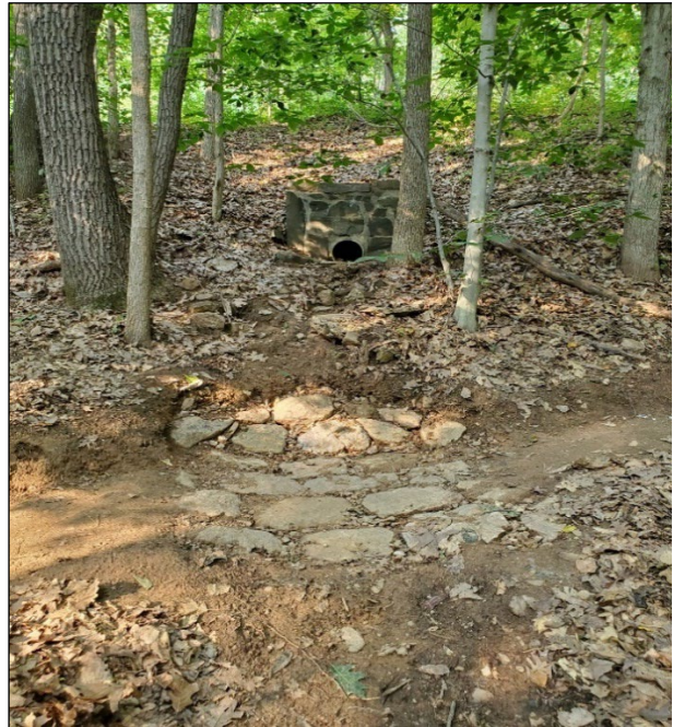
Armored swale in slight dip.
