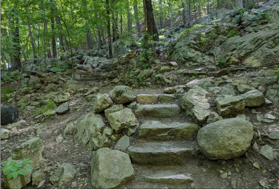
Short flights of stone stairs are a sustainable way to gain elevation on steep slopes, and when built correctly can last for many years with minimal maintenance.
