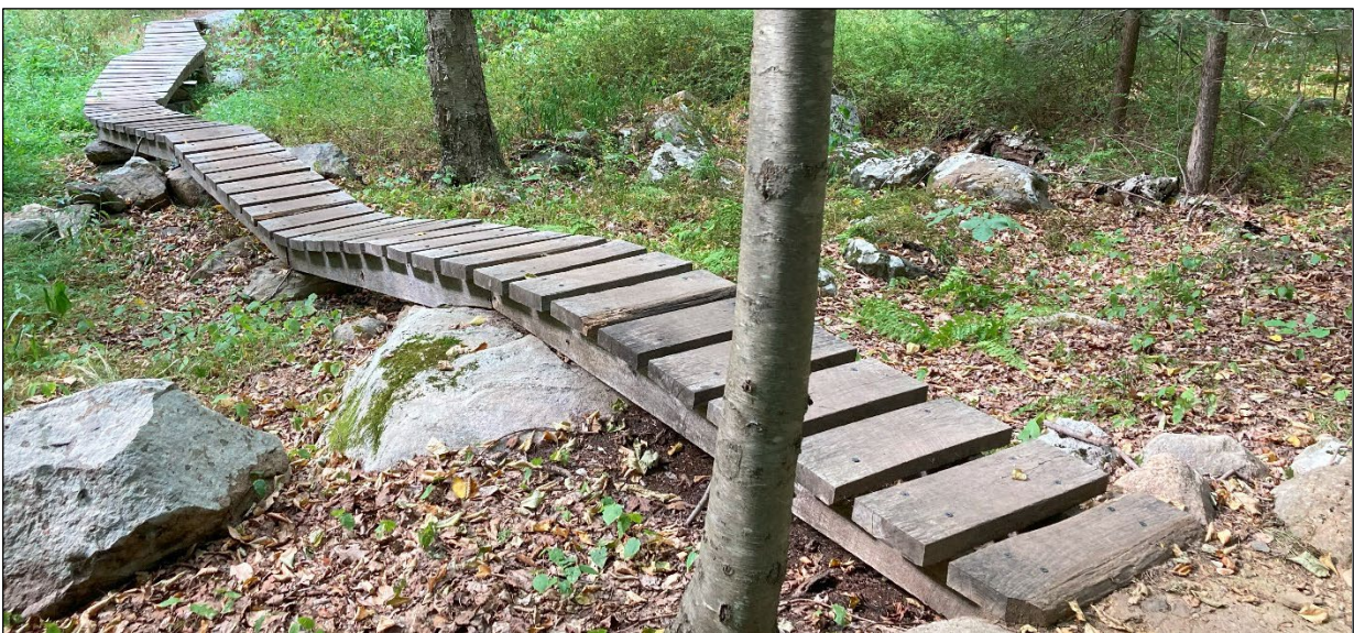
Boardwalks can use native stone as sills with the right pinning and mounting hardware, as seen in this creative mountain bike trail structure.
