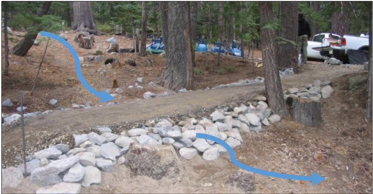
Capped drain lens, with arrows depicting where water flows downhill and passes through loose stones to travel under the trail.
