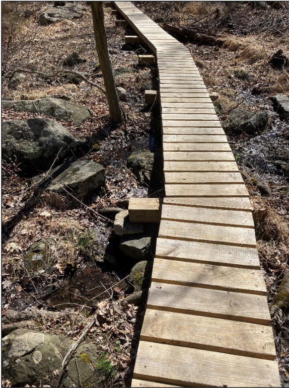
Simple, backcountry boardwalk showing how turns can be accomplished with planks cut at angles.
