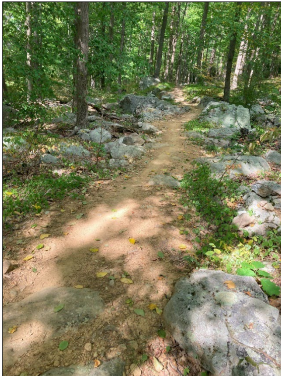
Local mineral soil is often used to provide a stable and durable surface.
