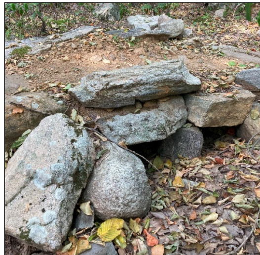
Closed and surfaced culvert.
