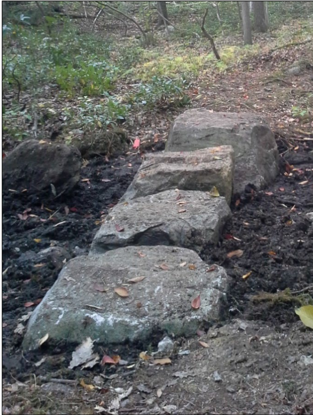
Two examples of stepping stones used to cross muddy ground.
