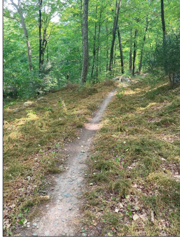
A narrow single-track multi-use trail, with a tread surface roughly 18" wide.
