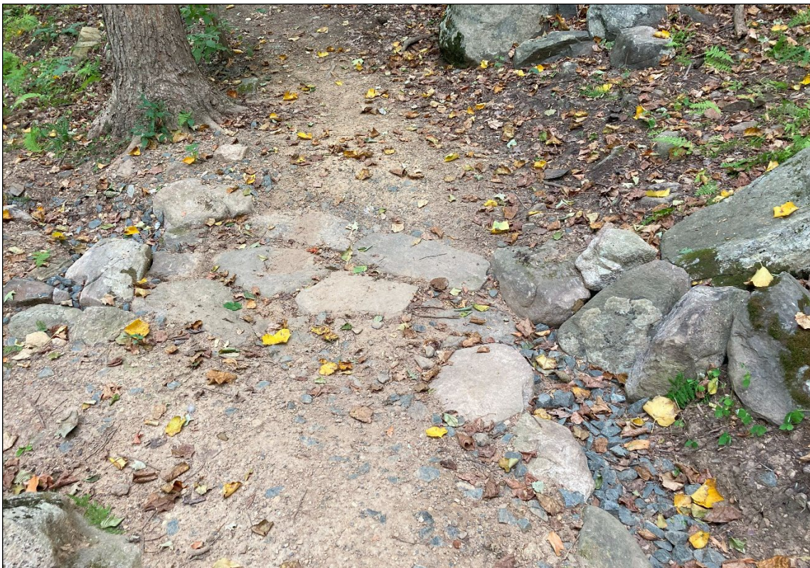
A small armored swale with gravel on the right side to slow water flow and reduce erosion. Note that this example, and the others on this page, feature loosely-space stones which yield gaps that would not comply with FSTAG standards.
