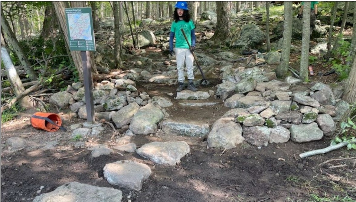
A series of stepping stones leads across a muddy area to a dry and firm landing.
